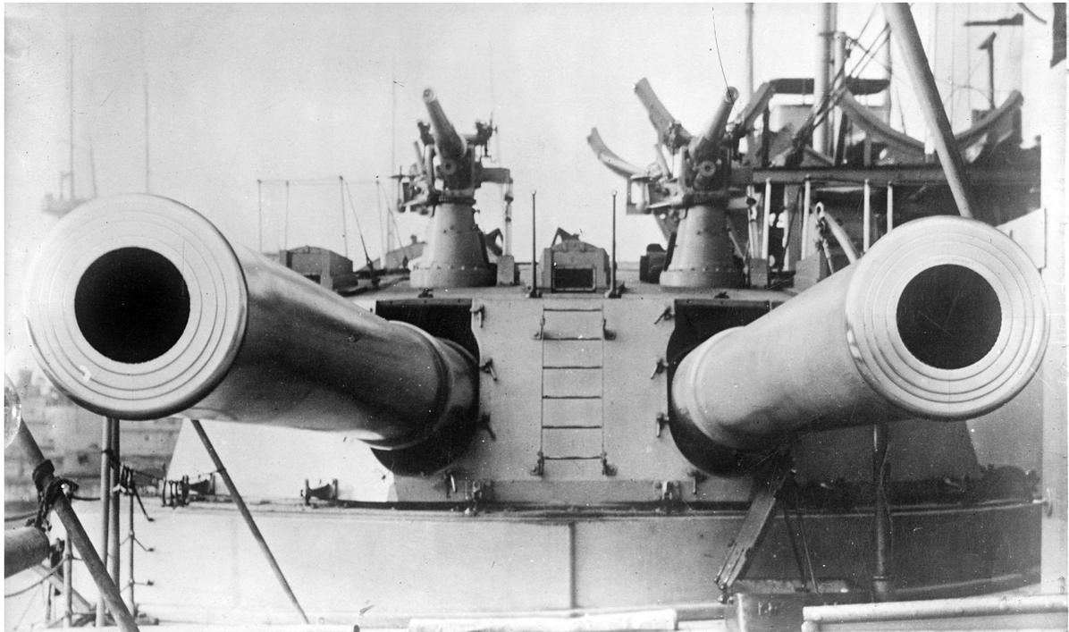
Figure 2: Turret with twin 12-inch Mk-X guns on HMS Dreadnought. <sup>12</sup>
